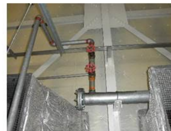
Riser pipe installed from above
