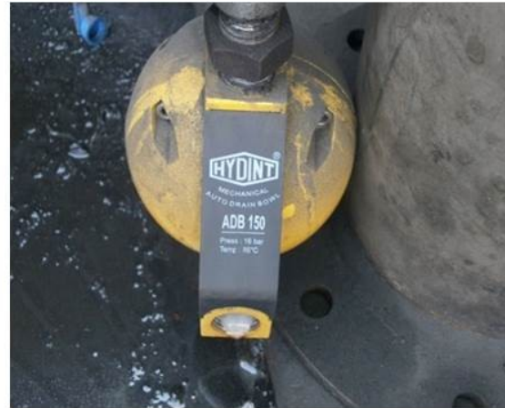
Automatic Drain Valve (mechanical type)
